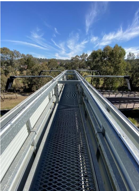
Photo 8 – General view of upper catwalk
