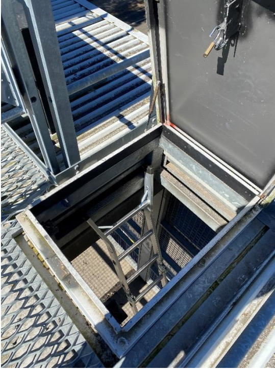
Photo 3 – Secured access hatch in roof of pedestrian bridge.
